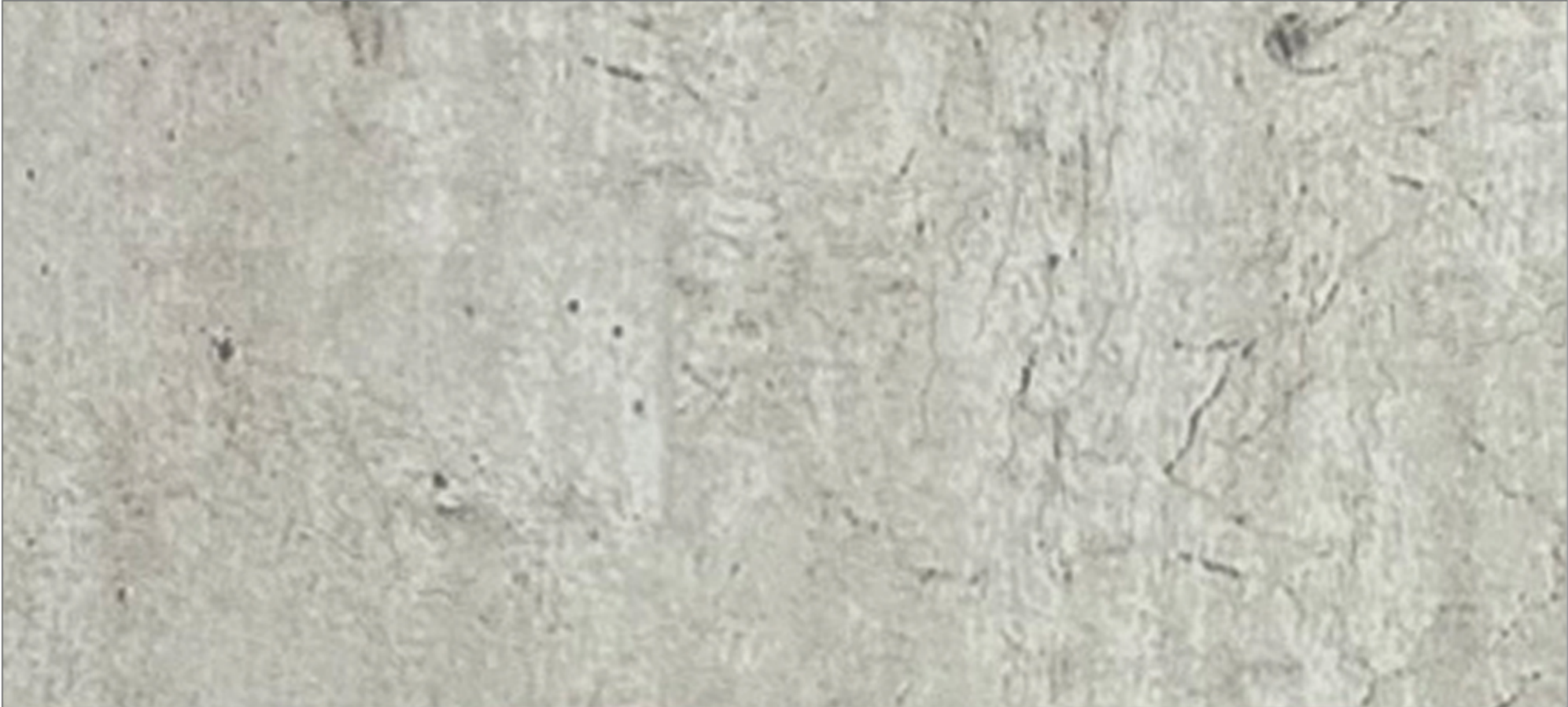
CN 6483 P Concrete
